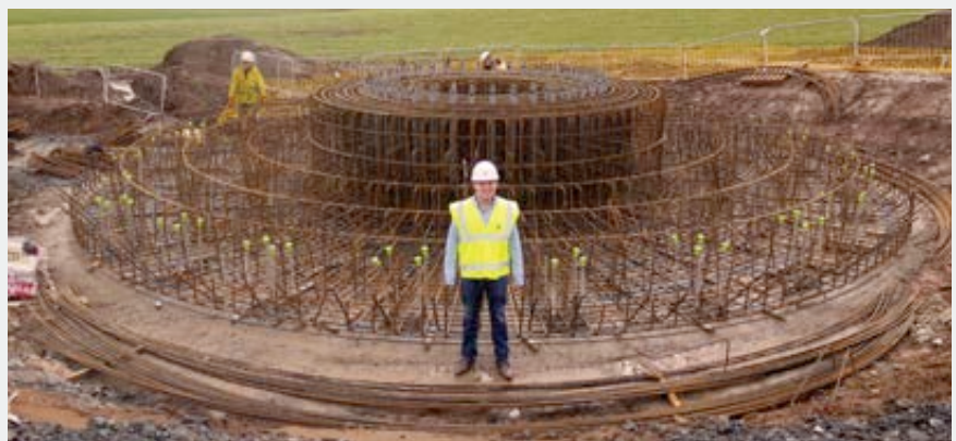
Wind turbine groundworks, Stewart Energy
